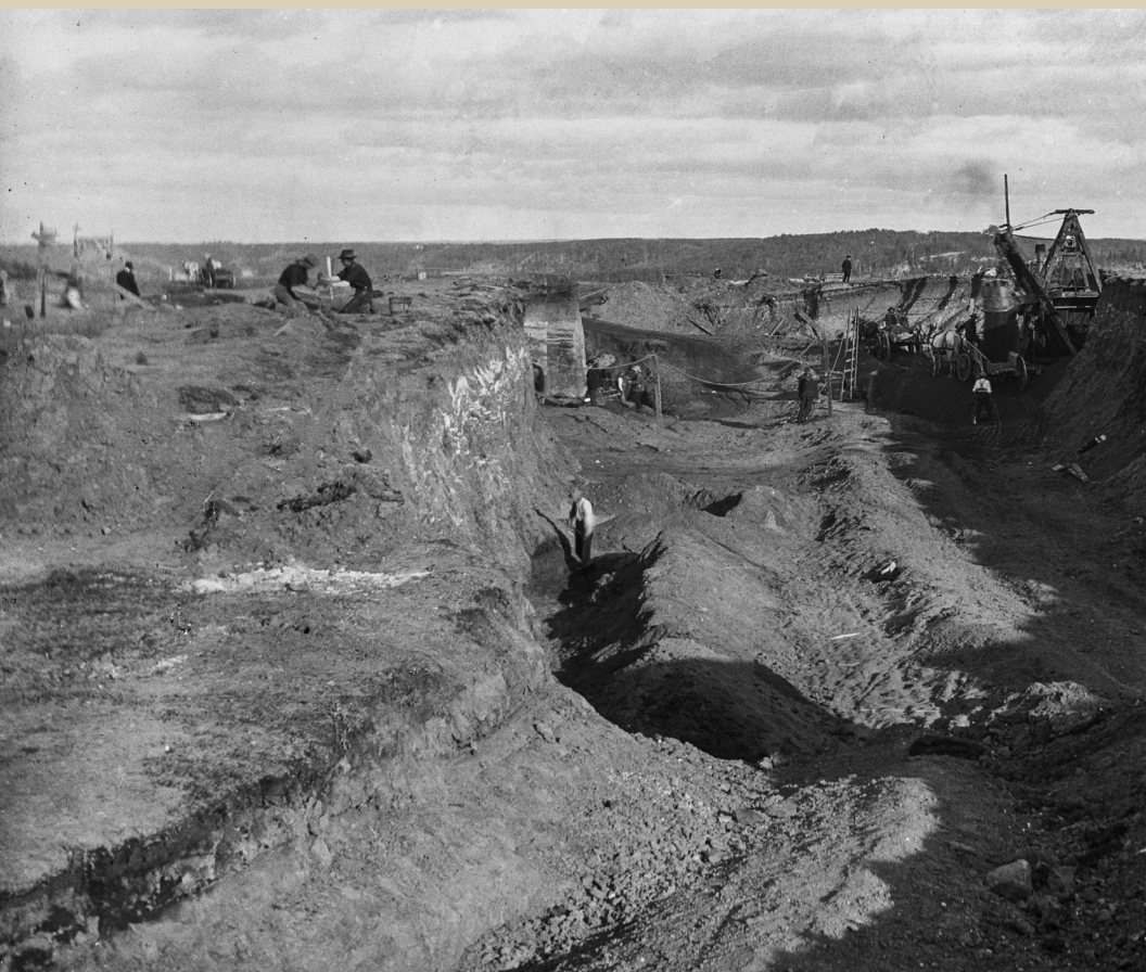
A steam shovel excavating for the Legislature Building, October 1907. PAA B3356
