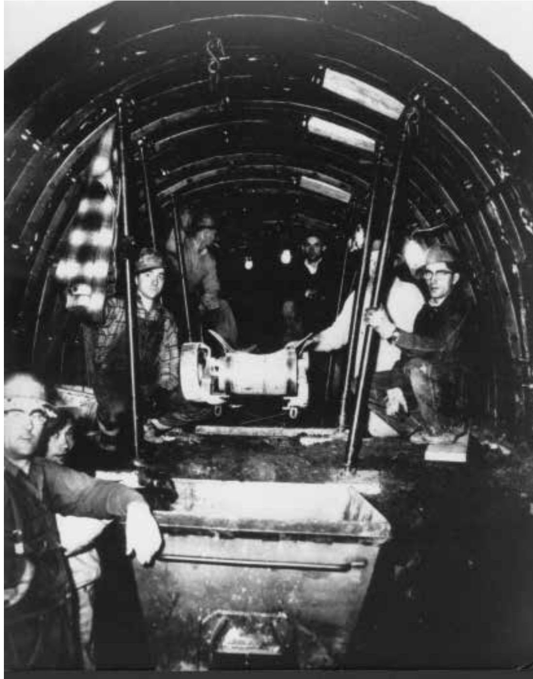
1950 National Union of Public Employees, Local 30 sewer construction workers. Sewer construction, like coal mining, is a dangerous occupation. Through the efforts of the union movement, it has been made safer.
