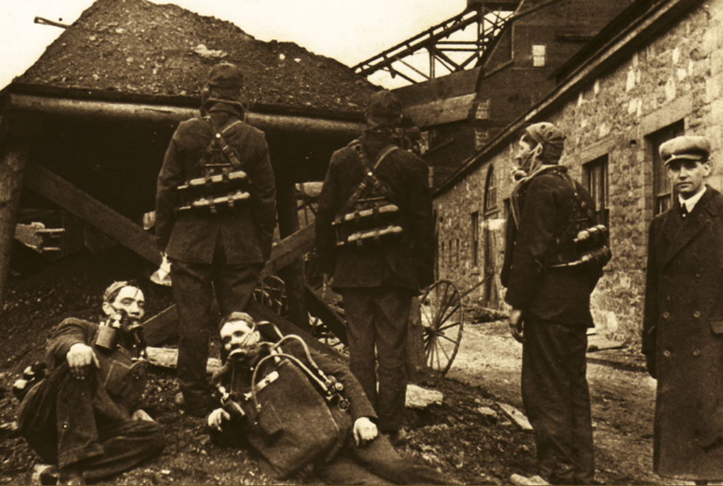
- Mine rescue team takes a break , Hillcrest, 1914
